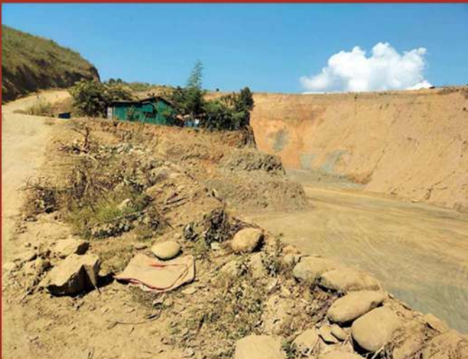
Figure 7 A picture showing how a village road was damaged and destroyed due to jade mining operations.
