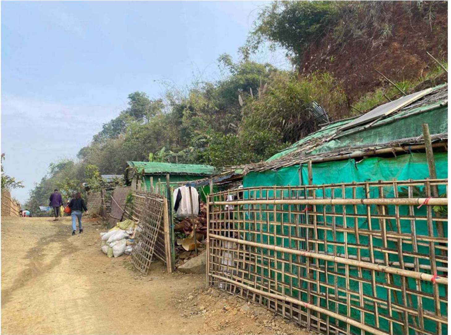
Figure 10 Following the forced displacement of Sabyit Hku villagers, they are now living in unsafe and precarious housing conditions.
