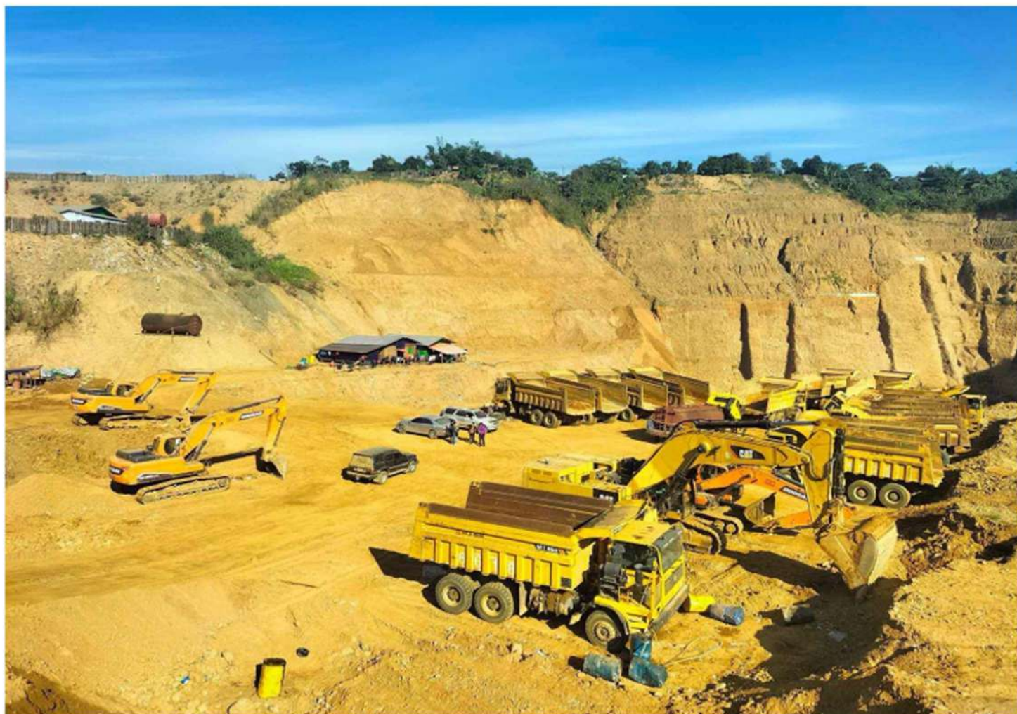
Figure 1 Excavation with heavy machines, such as excavators and trucks.
